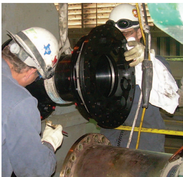
Figure 3. Installation of flexible disc coupling.
