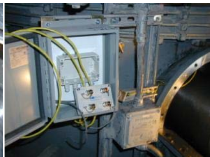
Sensor Terminal Box
