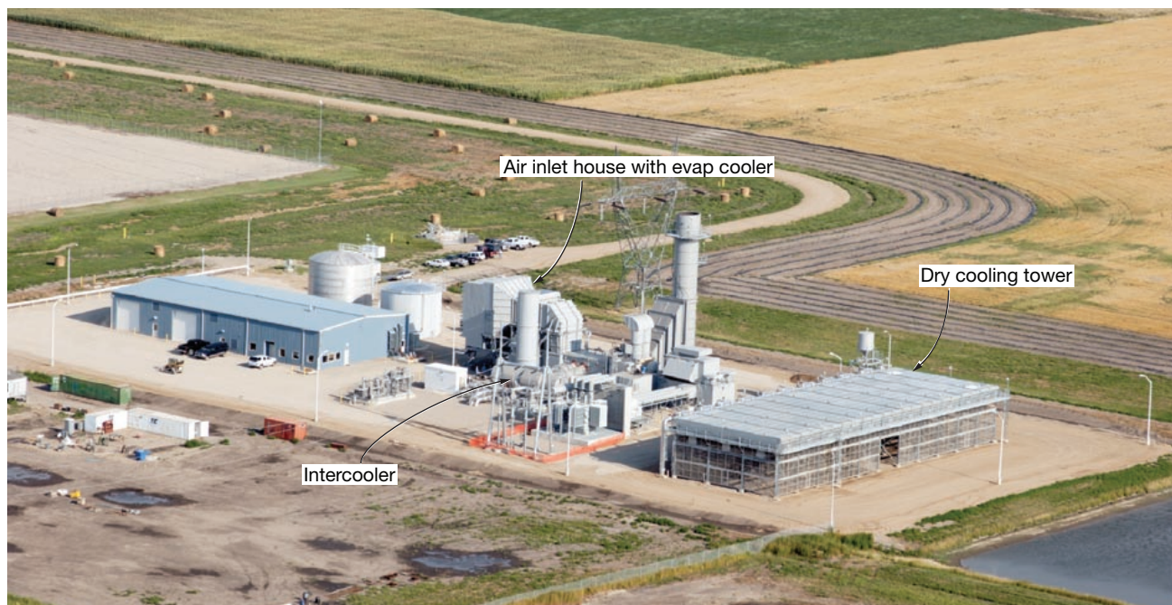
Basin Electric’s Groton Generation Station, site of the world’s first commercial LMS100, will begin installing a second unit this year and bring it online early in 2008
