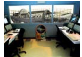
EXAMPLE CONTROL ROOM
